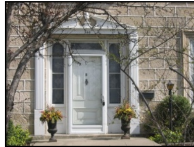
Janefield Entrance, 366 College Avenue, Guelph, c. 1854 (Canadian Register Nomination)
